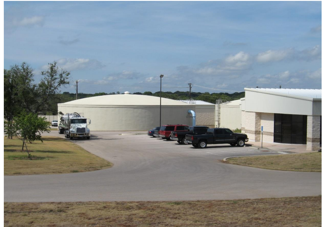
Storage Tanks / (2) 1 million gallon
