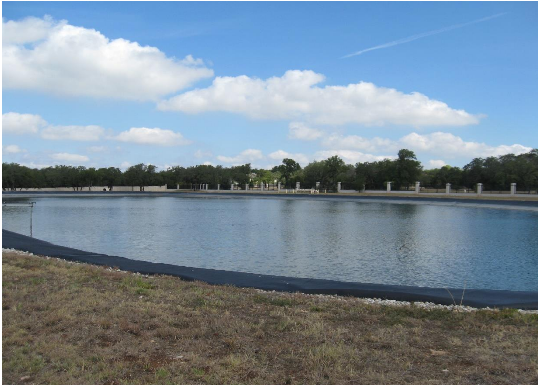
Raw Water Pond / 8 million gallons
