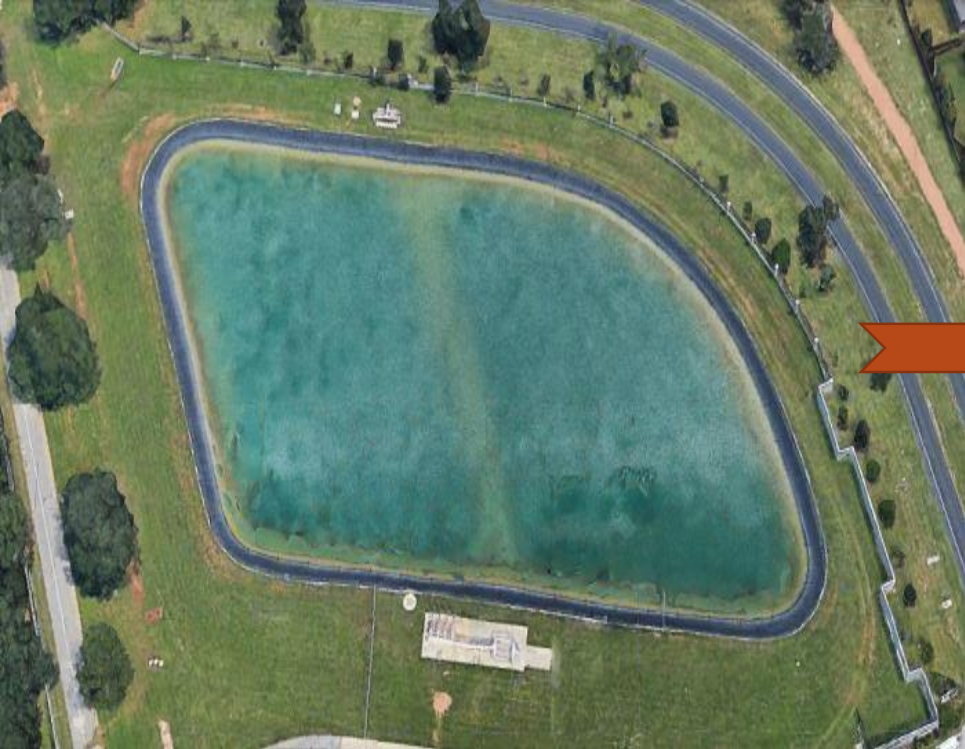
Raw Water Pond
