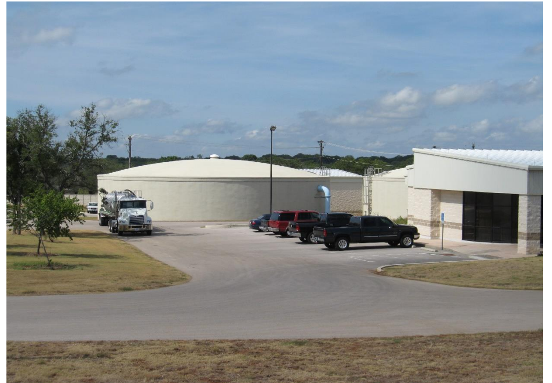
Storage Tanks / (2) 1 million gallon
